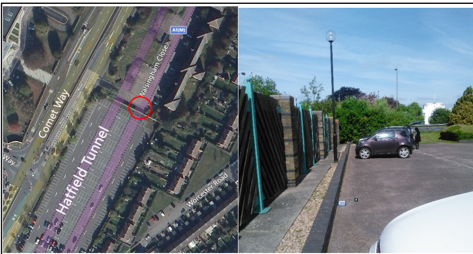
Figure 1 – Hatfield Tunnel Vibration Survey Location
