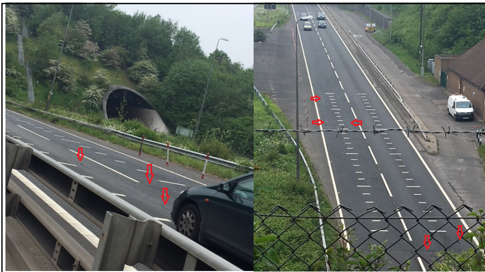
Figure 3 – A20 Road surface near vibration survey locations
